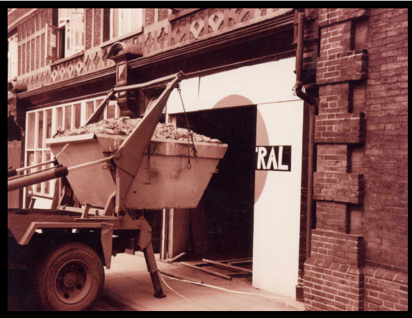
Plaster being removed
