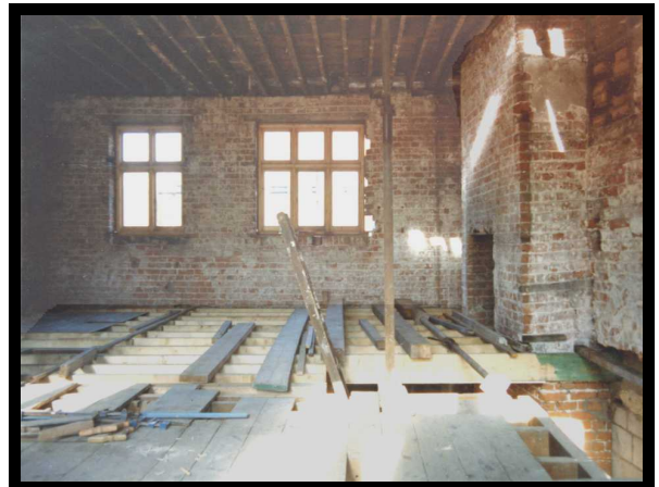
New timber joist to all levels
