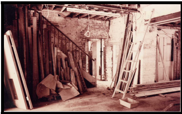
Staircase, joists, floors removed
