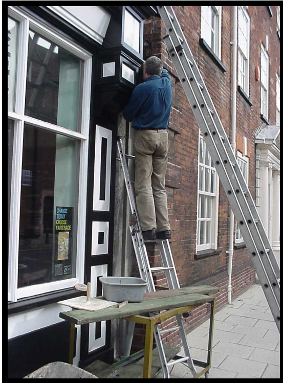
Restoration of the cornices and installation of double glazing to new shop front Marmolleum flooring with cork insulation below
