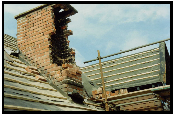
Rebuild chimney and waterproof the roof
