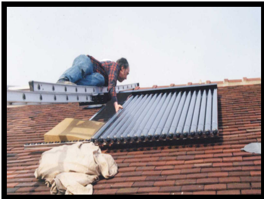
Solar tubes on 42-46 and 48
