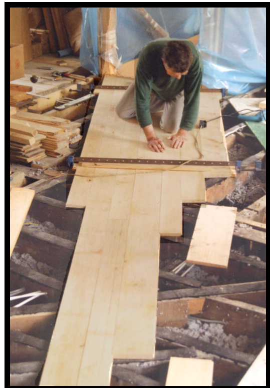
New timber floor to with cork and rubber below for (noise and heat) insulation
