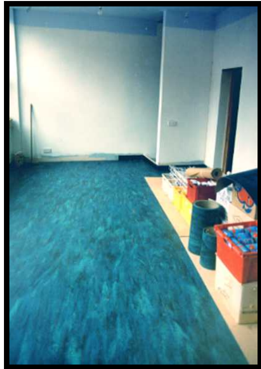
Restoration of the cornices and installation of double glazing to new shop front Marmolleum flooring with cork insulation below
